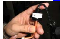
Figure 28: Pressostat de pression minimale.
